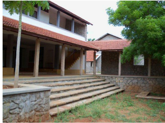
New Campus - Dormitories
