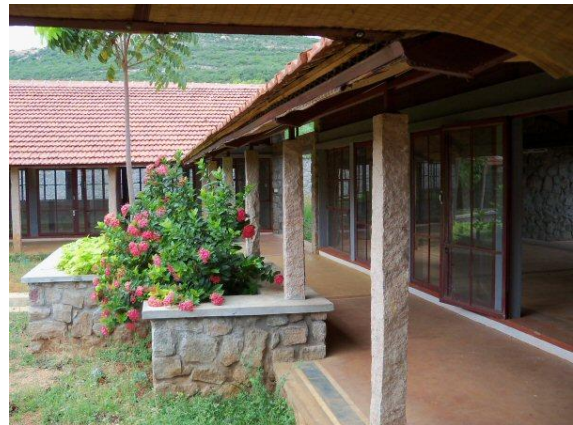
New Campus - Corridor
